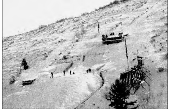
Gully between large takeoff and knoll of the underhill prior to regrading, early 1930
