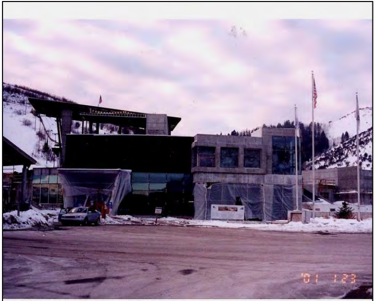
Joe Quinney Winter Sports Center / Alf Engen Ski Museum under construction, January 23, 2001
